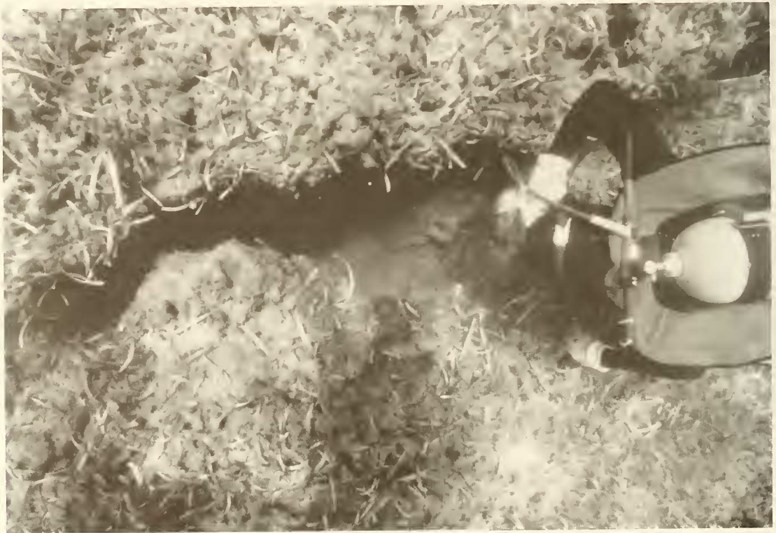
Figure 6. Initial crack prior to incipient fracturing and slumping.
